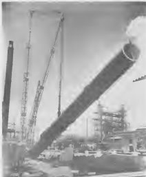
THE RING of holes at the stack's base was first positioned on the bolts on the east side and then skillfully slipped over the others. Below, the giant just she left her horizontal resting place.
